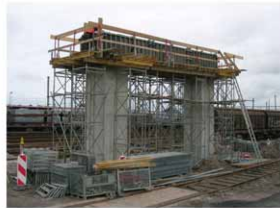
11 Stahlbetonrahmen in Achse 3 © Fritz-Dieter Tollé
